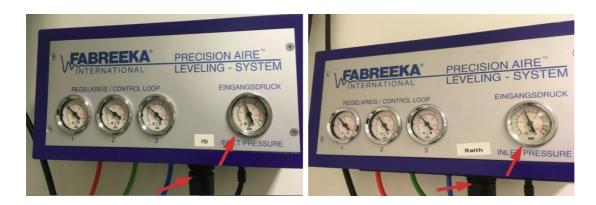
The vibration isolating platforms for the Raith 150 EBL and the FEI Nova 200 SEM/FIB are driven by an air compressor outside of the Nanolab. The compressor is located on floor zero of the Albanova main building. The incoming pressure should be around 9 (7?) bars, this can be regulated with the black knob on the underside of each control unit.
