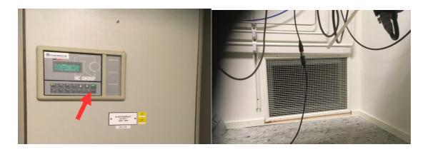
Check if the ventilation controller is on. The ventilation unit is located in the Ebeam-service room. Switch on if it is off.
