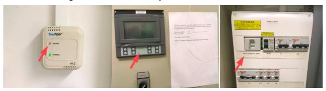
This was solved just by switching off and on the main switch on the controller. The controller is located in the small room between the AFM lab and the Deposition lab. The controller cabinet in the center picture must be opened to reach the mains switch (right picture).
