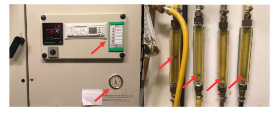
This is the cooling water unit in the service for the Ebeam and the Deposition labs. The controller usually shows an alarm (silent), it does not stop after a reset (red arrow to the top left).
